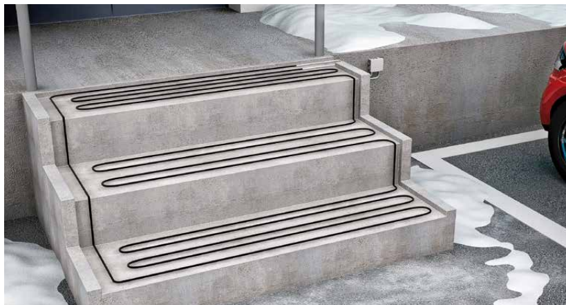
Tash constant wattage cables are always installed into a loop and the conductor is always connected to the junction box with a cold lead. (THE PICTURE IS AN APPROXIMATION)
